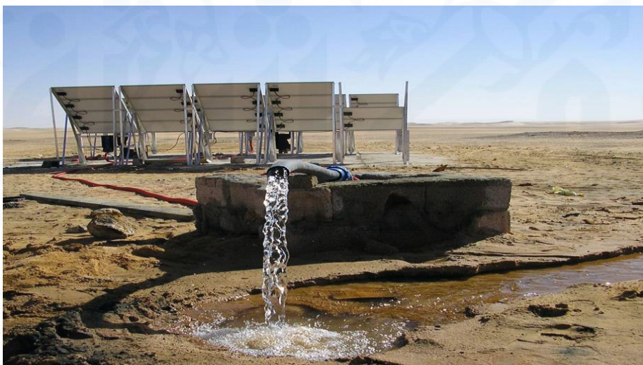
Figure 4.17 PV Water Pumping Beer Tssawa Source: Mohamed Ekhlal et al 2007
